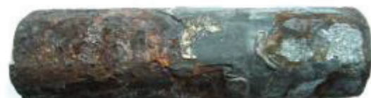
Figure 11 - Severe Corrosion on the Surface of the Inner Sleeve [1]
