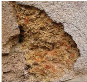
**Figure 4 - Soil erosion in House 15 (Base of external wall)**
