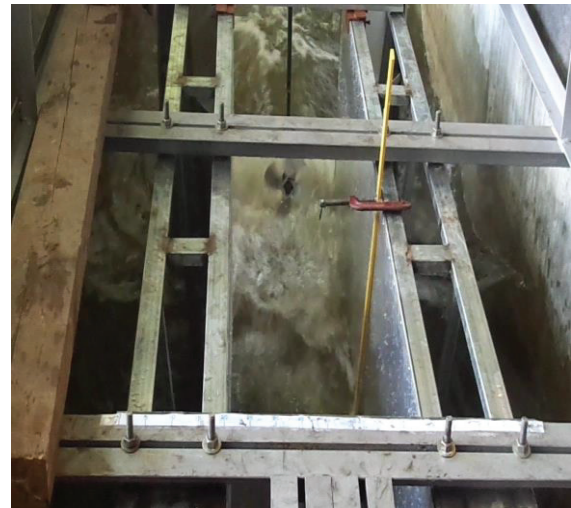
Figure 3 - Turbine placed at the channel end
