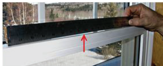
Figure 1 - Deformation in a Al 6063 door frame
