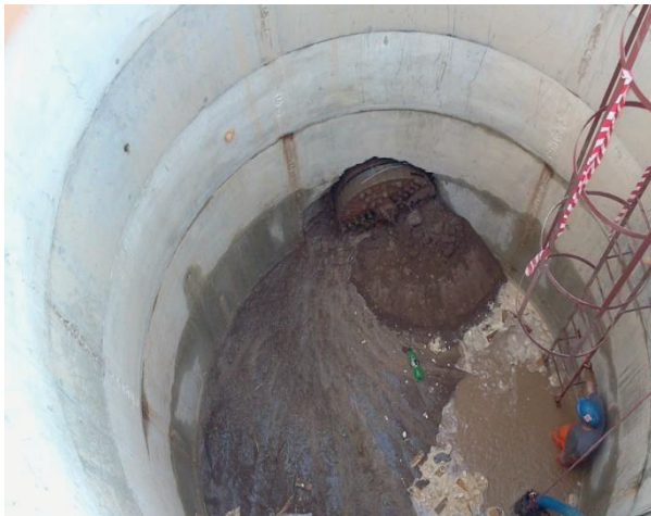
Figure 1 - Micro tunnelling machine emerging from the exit shaft
