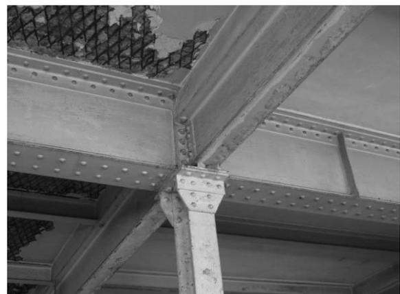
Figure 1 - Exposed steel columns and beams in the 125 year old Gaffoor Building
