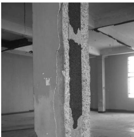
**Figure 2 - Significant corrosion in concrete encased steel internal column in Central Point building**
