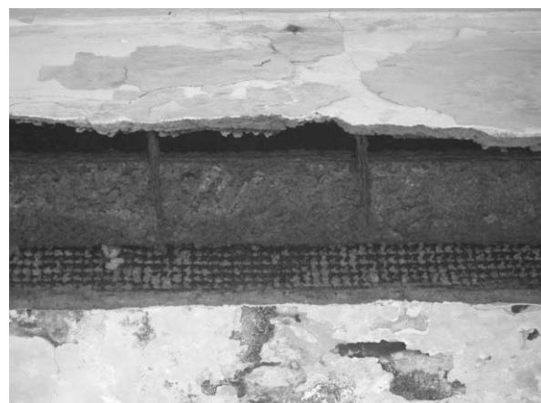
**Figure 3 - Corrosion in steel floor beam covered by wire mesh and plaster in Central Point building**
