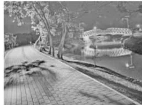
Figure 7- Paved section of the foot path
