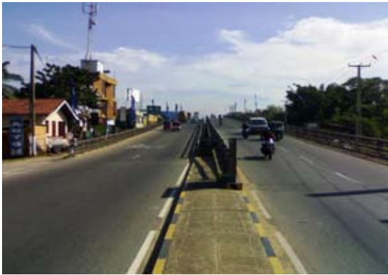
Figure 2 - Pattiya Junction Flyover along A01
