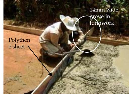
**Figure 3 -Construction of half depth contraction joint**
