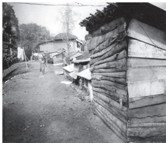
Figure 3 - Encroachments, Kelani Flood Bunds
