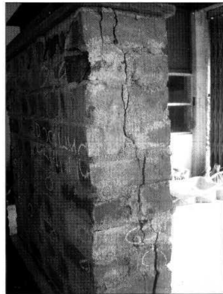
Figure 10: Tested brick panel
